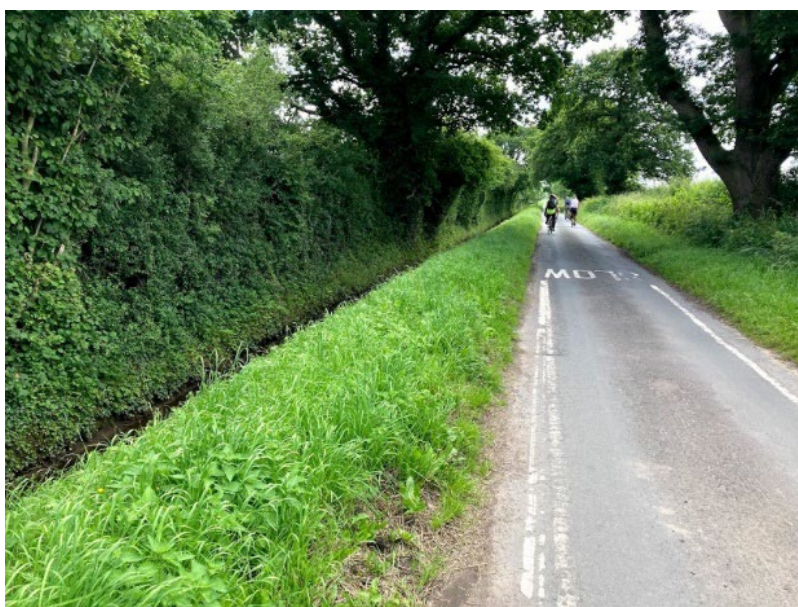
Figure 9: Langwith Stray – a narrow carriageway bounded by drainage ditches and high hedges, Sustrans 2022
