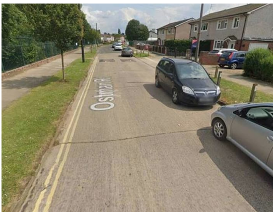
Figure 6. Concrete Slab Surfacing
